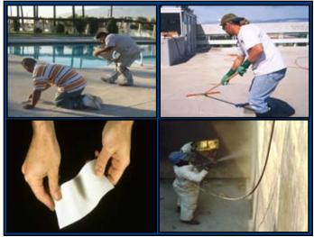
MPC can be flexed through 90° angles without cracking or loss of adhesion.
